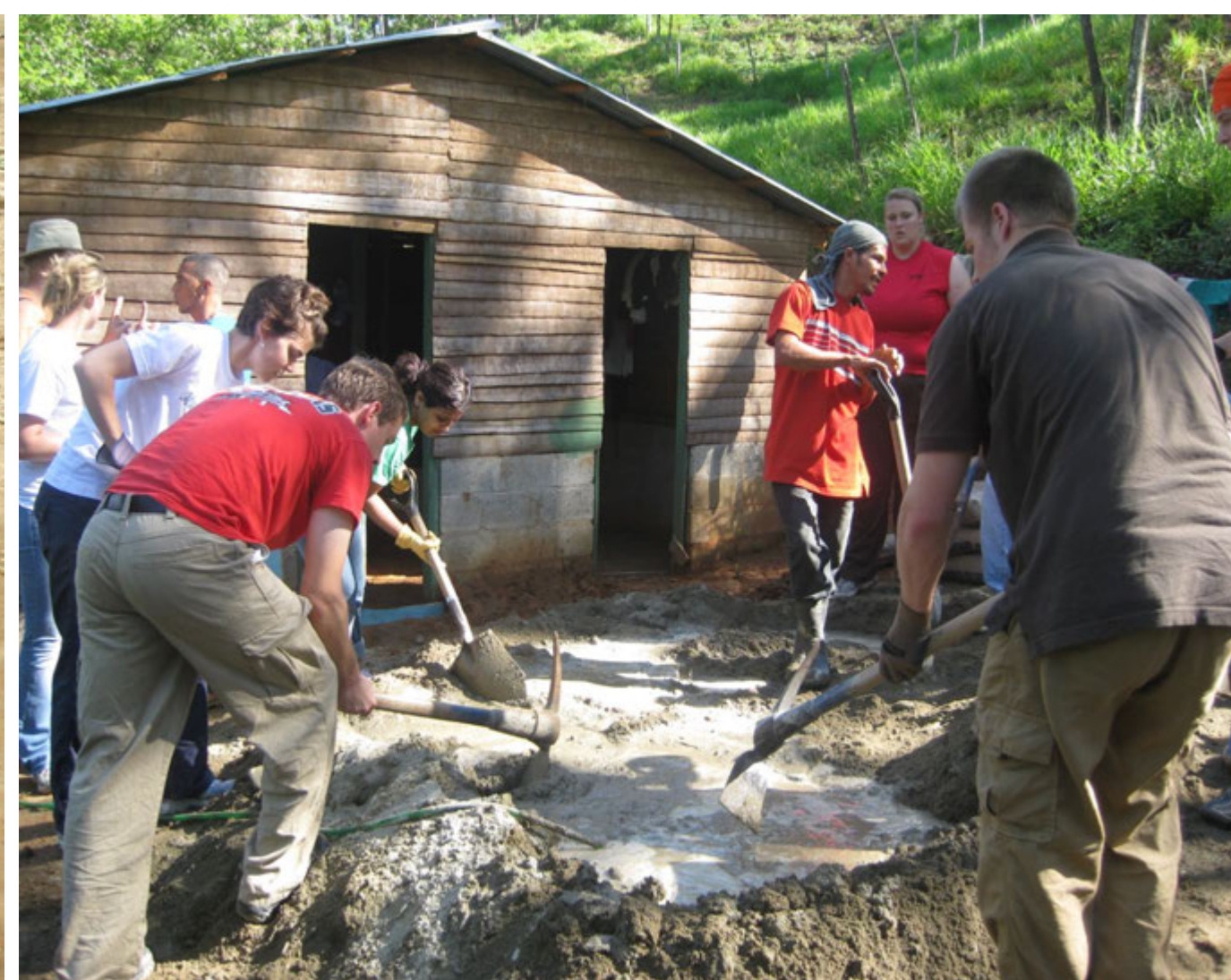
Participants laying concrete that will replace a dirt floor in a family's home. This provides the family with a sanitary and permanent living space and the opportunity for a more healthy lifestyle.
